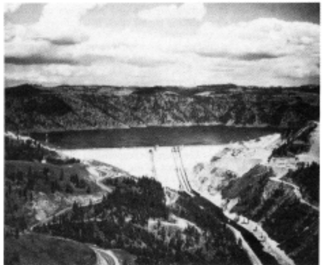
The power-generating capacity of the multipurpose Dworshak Dam in Idaho is currently being expanded
